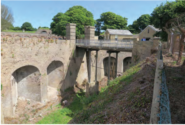
Burgoyne's 20C entrance bridge, the four flanking casemates below. Photo Clive Penfold
